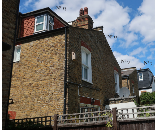
From rear garden - Back of terraced houses (Davis Road)
