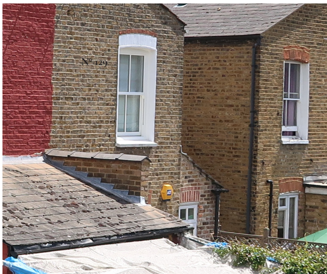
129 St Elmo Road - Side return extension
