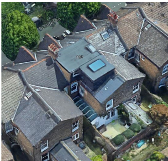
119 St Elmo Road - Side return extension
